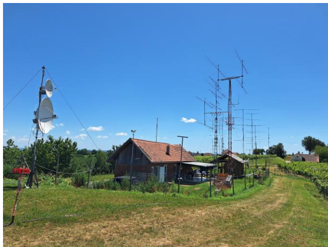
Part of S59P's multiband antenna system. During high-rate periods, operators divide the receive antenna systems so they can listen in several directions at once.
